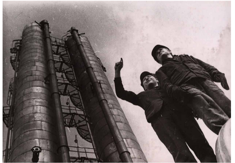
"Distillation Columns for Methanol Production at the Shchekino Chemical Combine (1957)" Gosudarstvennyi arkhiv Tul'skoi oblasti f. P – 3986, op. 7t.5, d. 1865, (no pagination).
